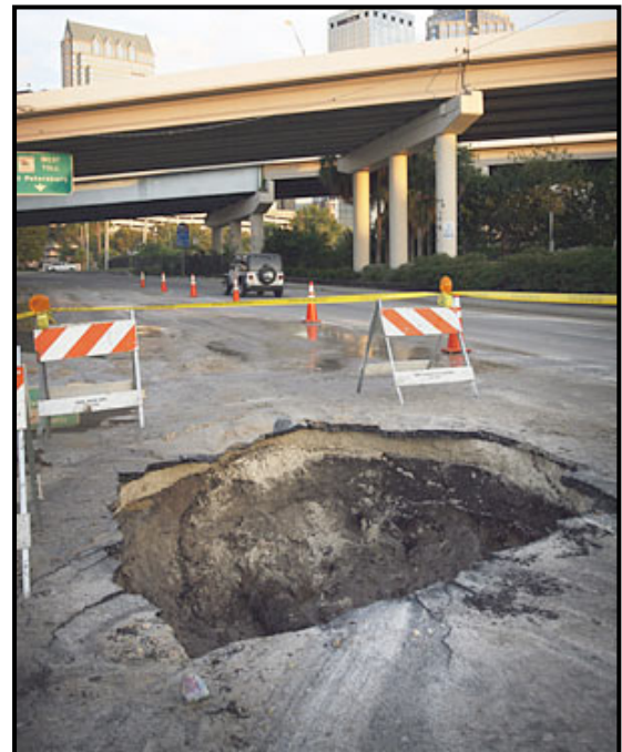
Sinkholes can appear suddenly and cause significant damage to infrastructure.
